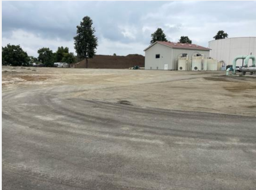
Figure 3. View of water tank within Project area, view facing northeast.
