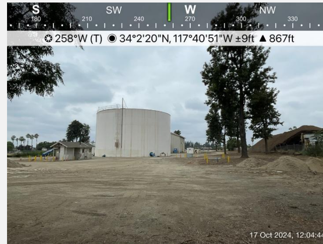
Photo 2. Overview of site, taken from northeastern corner.
