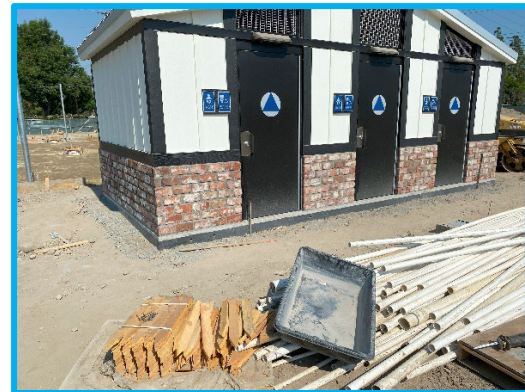
Restroom with wainscoting installed.
