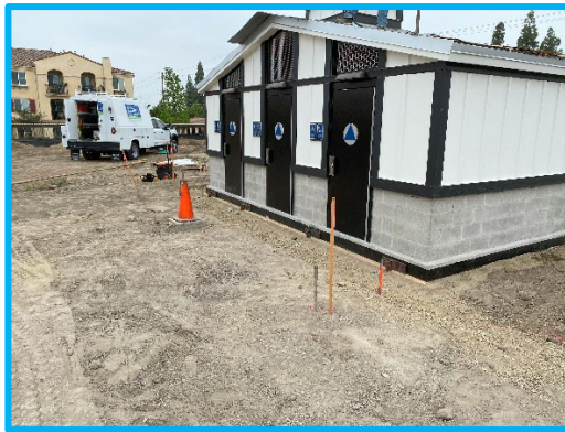
Restroom when delivered.
