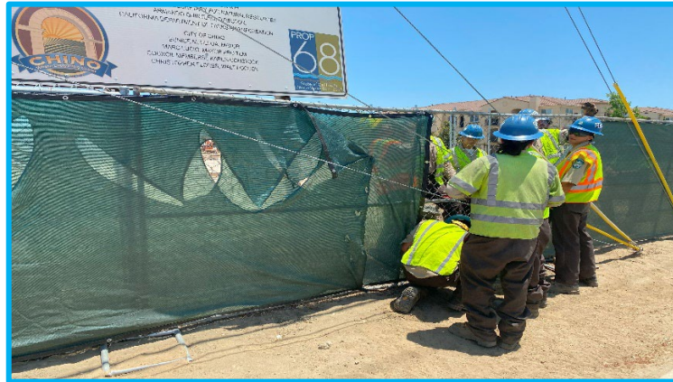
CCC members working on site.
