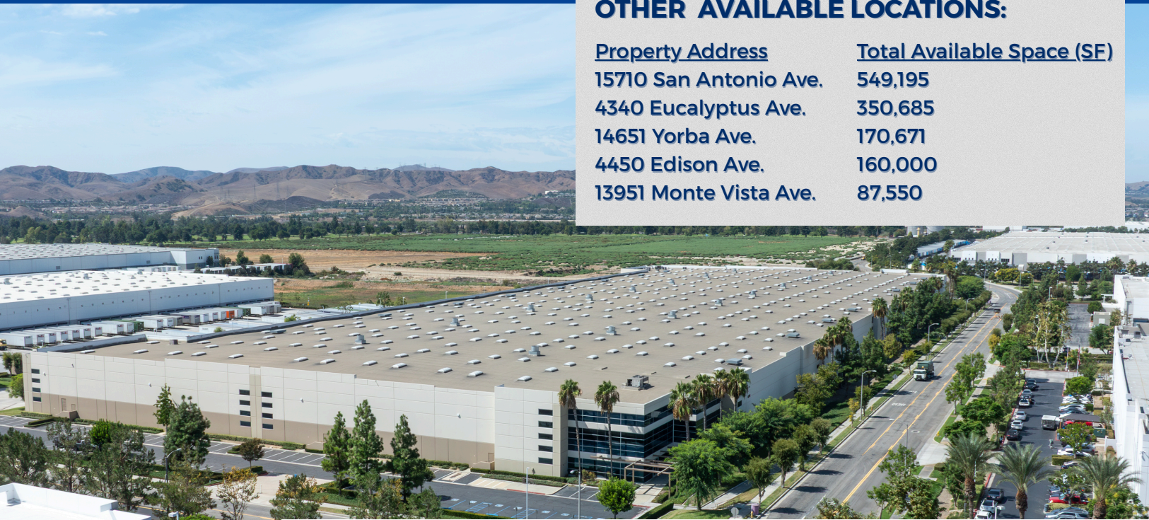
6711 Bickmore Ave - Chino South Business Park Distribution
