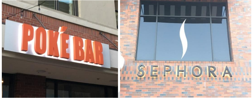
Figure G. Examples of pan channel letters and internal halo illuminated channel letters in wall mounted signs
